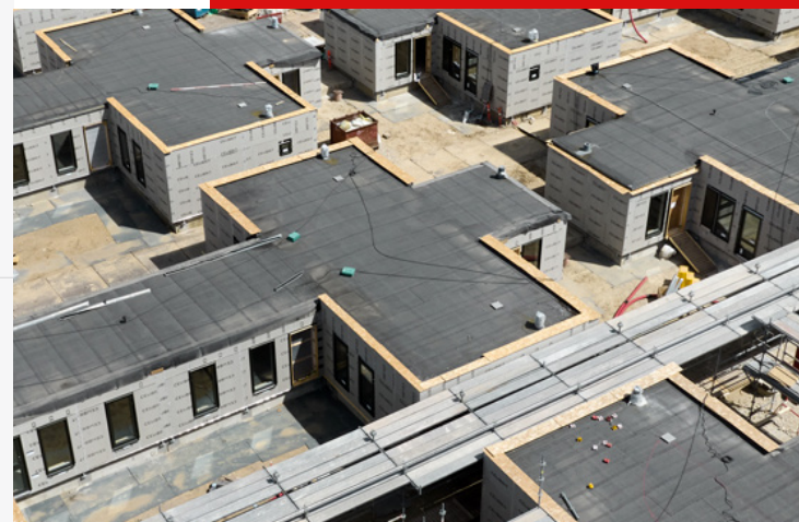
< RENOVATION OF GALGEBAKKEN
